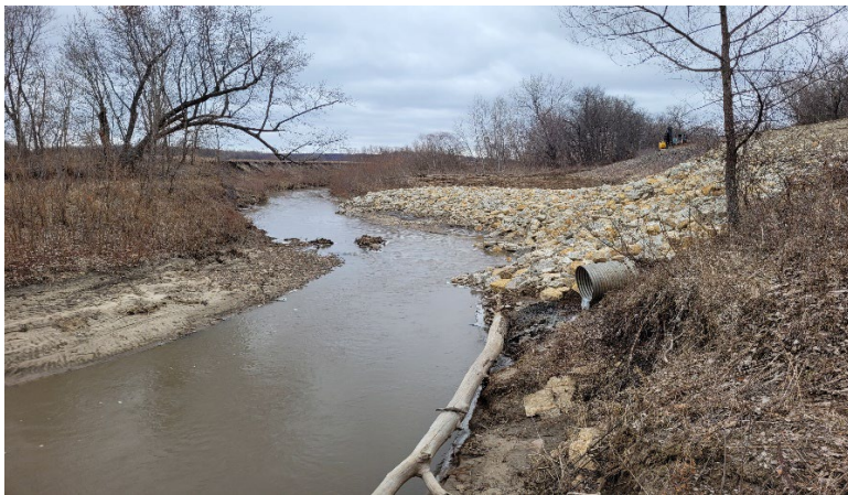
Stream bank repair for erosion in Decatur County
