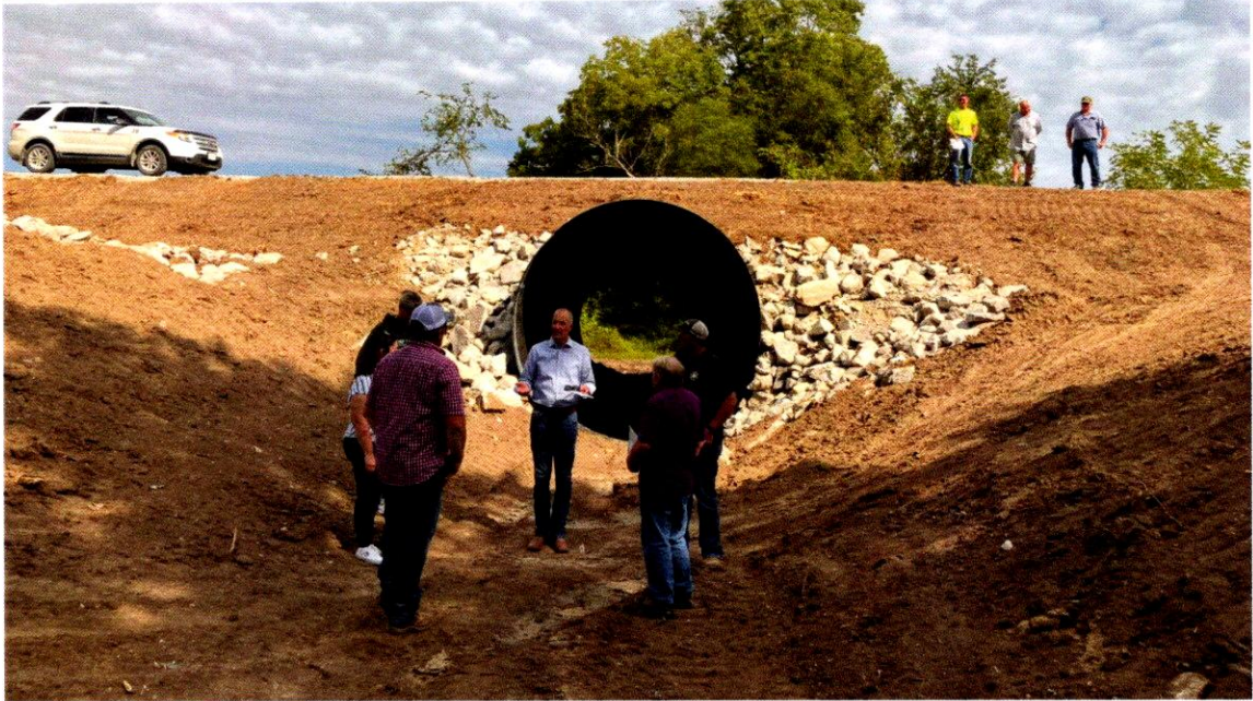
Sec. Naig visit at a SIDCA bridge replacement in Davis County
